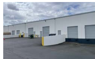
3 GRADE-LEVEL DOORS & 2 DOCK-HIGH DOORS
