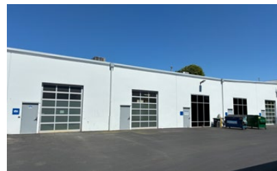
3 GRADE-LEVEL DOORS (2 MORE POSSIBLE)
